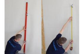
4. Measure and mark places for installation of the remaining brackets.
