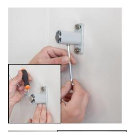
Loosen clamping screws, then pull out bracket bolts.
