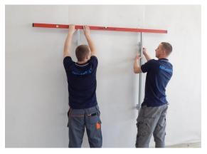
Set the level of upper edges of installed guide rails.
