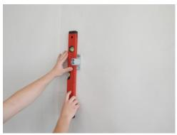
3. Check levels of the brackets, if needed correct it and secure the brackets
