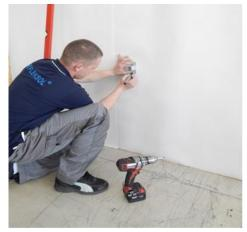
Designate spots in the axis of installation of brackets to the base. Put the bracket on the base and mark places for installation holes.
