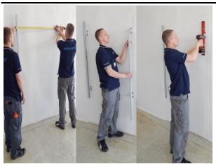
Use measure tape and spirit level to transfer installation places for second guide rail.
